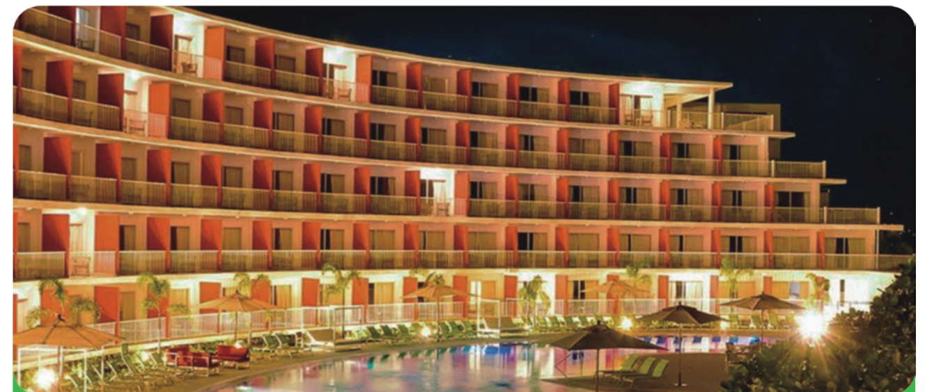
Montego bay resort in Jemaica, with DC inverter VRF system.
